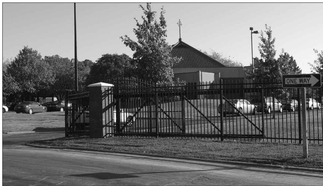
A new fence has been erected at Bishop Kelley High School.
