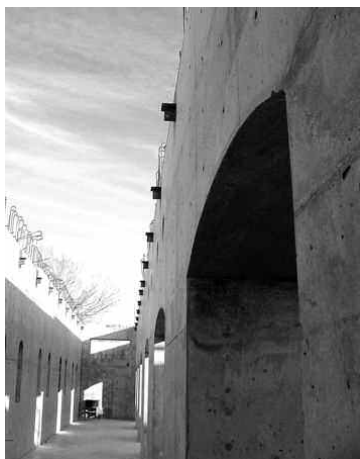
A view of the inside of the crypt's north wall.
